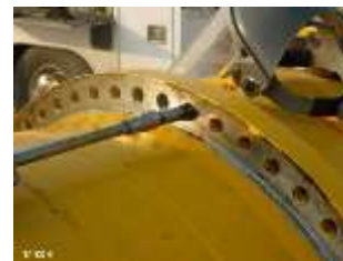
Cleaning paint and rust prior to torquing
